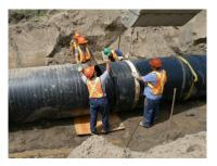
At the joint, apply a heated Wehoseal membrane to prevent grout infiltration. See the instructions for the installation of the membrane in the annex.
