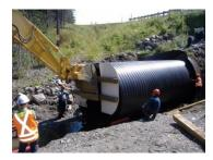
8. Sections can also be inserted by pulling. For a pipe with restrained joints (screwed or welded), bolt the plates at the end where you pull. For a pipe with unrestrained joints (bells), install the cross in the bell of your last pipe.
