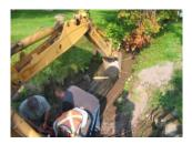
4. Lay the first section of pipe in front of the pipe to be rehabilitated, the male end towards the inlet. Readjust the seat if necessary: the alignment between the new and the old pipe must be perfect.
