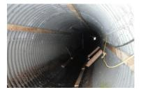
6. If the injection is to be made using parallel pipes, these should be attached to the new pipe as the insertion proceeds. Provide a pipe for each casting.
