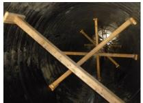
12. Proceed with grouting, respecting the number of pours specified in the following table. If more than one pour is necessary, allow it to set for at least 12 hours before pouring the next one. The pipe should be carefully monitored and if necessary, internal bracing should be installed to restrict any deflection to this limit.
