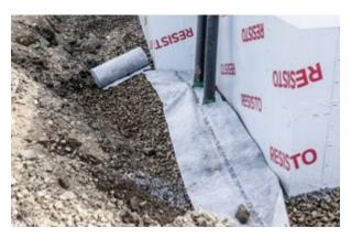
regular maintenance, a visual inspection by camera made easy by the green interior of SoliFlex and a pressured water cleaning will dilute the possible accumulation of ferrous deposits inside the drainage system, without damaging the surrounding soil and landscaping. Pre-assembled in the factory, the drainage access chimney is easy to install and ensures the system's sustainability.
