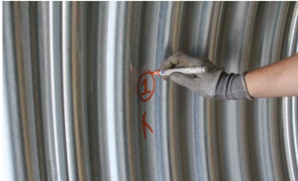
6c. Using the indelible marker, mark and number the position of the weir using the previously marked alignment line.
