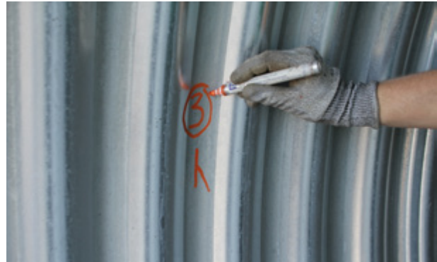
6d. Measure, mark and number the locations of the following weirs, following the steps mentioned above.
