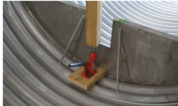
Note 2: Make sure you have a support (2x6 wooden suggested) to provide a stable base for your hydraulic jack.
