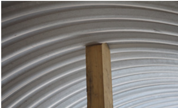
Note 1: Make sure your adapter has a beveled end so that it fits well in the corrugation.
