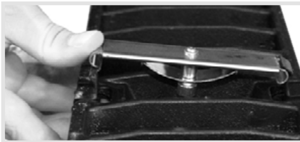
3a. Insert the vandal-proof lock under the grate.
