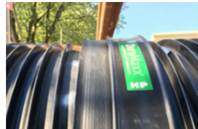
Completed joint insertion
