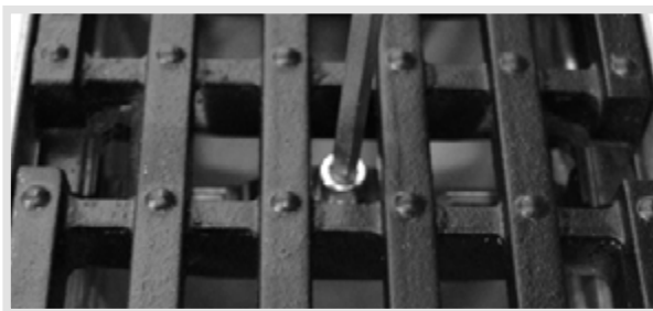
3e. Using a 5-mm Allen wrench, tighten the screw to expand the lock and thus prevent removal of the grate.
