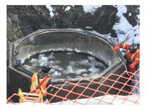
• For CDS-10 (octagonal shape), align the alignment arrows of all sections, while respecting the position of the inlet(s) and outlet.
