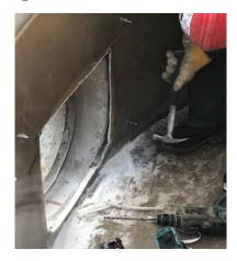
11. Apply a bead of polyurethane elastomer (butyl seal) and complete the sealing with Sikaflex 1a to seal the space between the fiberglass and the wall of the concrete structure of the manhole.
