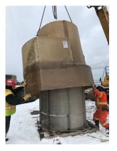
6. While holding in place the fiberglass separation cylinder (with the crane or power shovel), position yourself below the fiberglass part. Adjust the two elements, drill a first hole in the fiberglass and bolt the separation grid onto it. Make sure the separation screen is always centered before moving on to the next hole. Securely tighten the bolts and lock washers.
