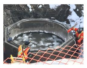
• For CDS-10 (octagonal shape), align the alignment arrows of all sections, while respecting the position of the inlet(s) and outlet.
