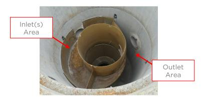
9. Cut the fiberglass at the inlet openings. Pay special attention not to damage the fiberglass floor.
