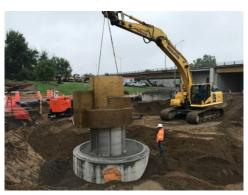
8. Position the inlet area of the assembly towards the inlet openings, while making sure to press it against the inner wall of the manhole.
