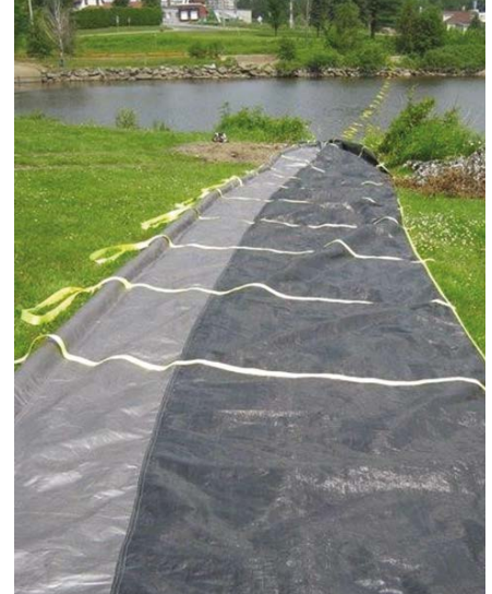
*Photo credit: Terraquavie
