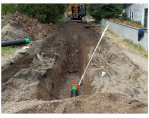
To effectively meet the specific needs of the city, the corrugated catch basin was punctured on the first top 12 rings to allow a second infiltration into the outlet and thus lower the water table. A custom frame was also installed to allow the installation of a pyramid grate, the standard used in the city's specifications.
